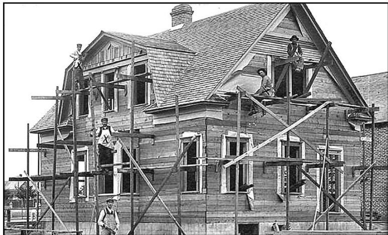
A typical Lauman Co. home, S.E. 22nd & Yukon, under construction, October, 1927. Using his wife's inheritance, Charlie built the house, intending it as a retirement home. They mortgaged it to cover other debts when the housing market collapsed, and subsequently lost it.
